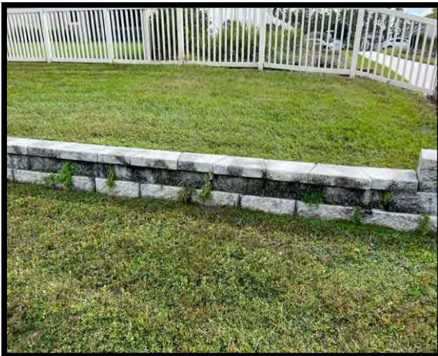
Footpath Retainer Wall: Spray for weeds and clean the wall.
